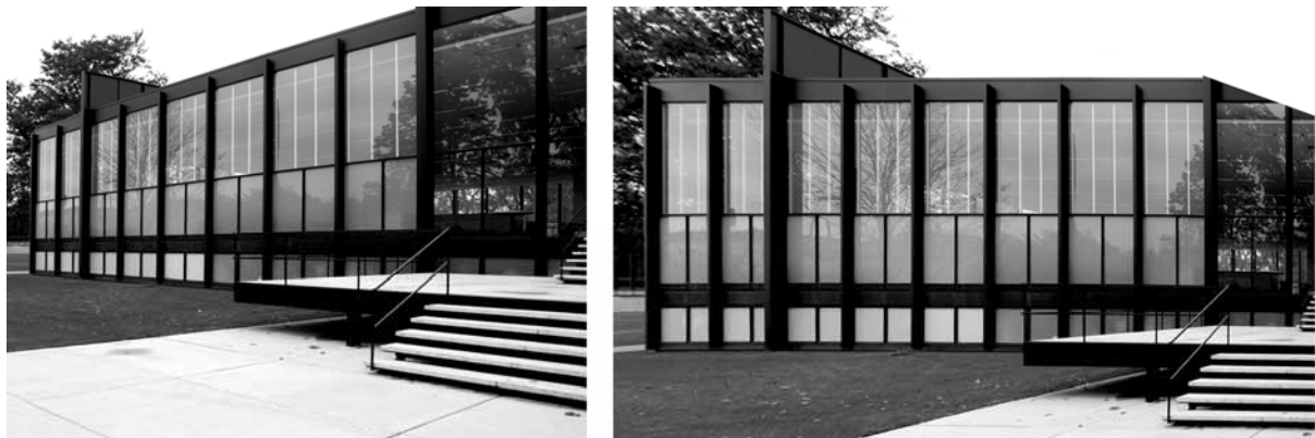
Figure 1. Crown Hall, Illinois Institute of Technology, Chicago, Illinois.
