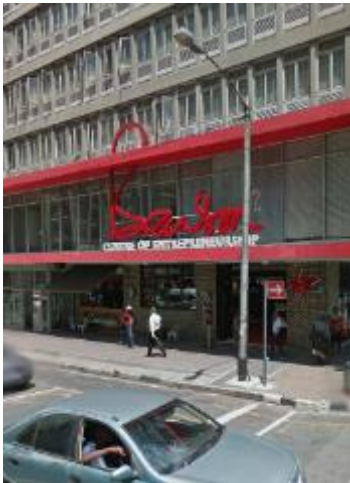
Figure 13: Branson building, often used by users to orientate themselves (Google Maps 2015)
