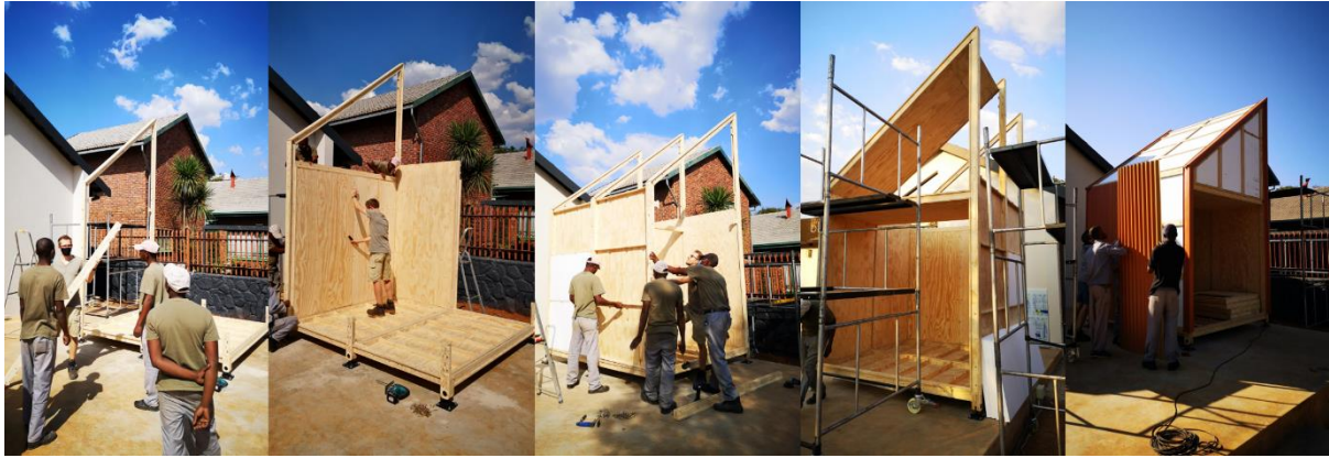
Figure 6: Rapid assembly of prefabrication components for Kospaza (earthworld Architects n.d)
